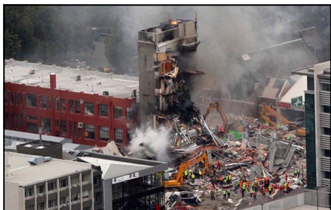
Figure 7. The Canterbury Television building in Madras Street, wrecked and then on fire after the earthquake (photo: Mark Mitchell).
